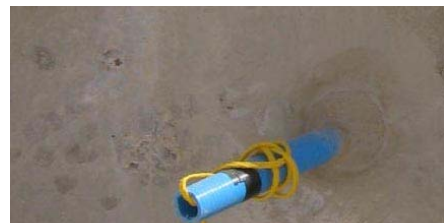
Trenches are created in the backfill for the slotted PVC conduit to be positioned and a hole is formed in the ring wall
