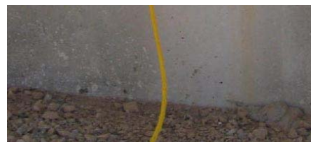
Slotted PVC conduit with a pull rope ready for the installation of the TT5000 sensing cable
